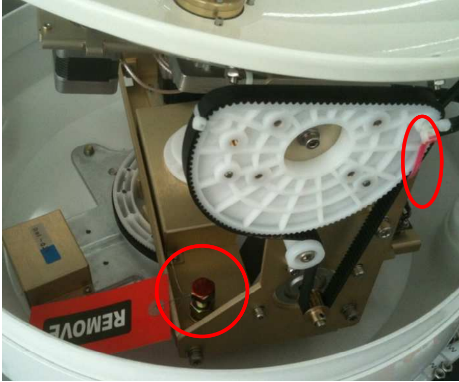
Figure 2-8 Fixed the Forms and Wire Ties
